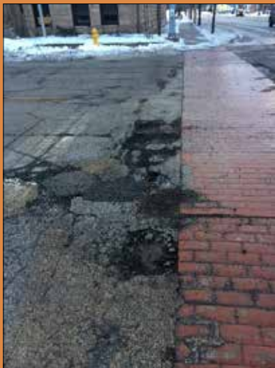
Figure 4.7 – Example of Poor Pavement Conditions, Rock Island, Illinois Due to Freeze/Thaw Conditions
