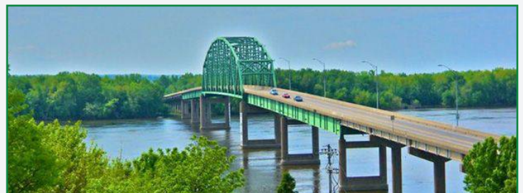
Norbert F. Beckey Bridge
