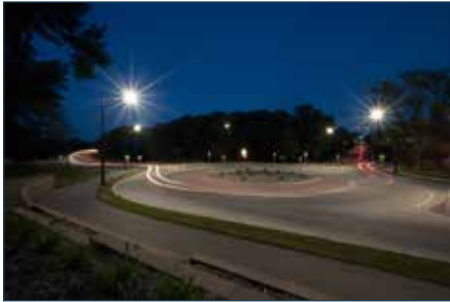
Roundabout used for traffic calming, crash reduction and energy efficiency by reduction in the use of signalized intersections which adds up to cleaner air.
