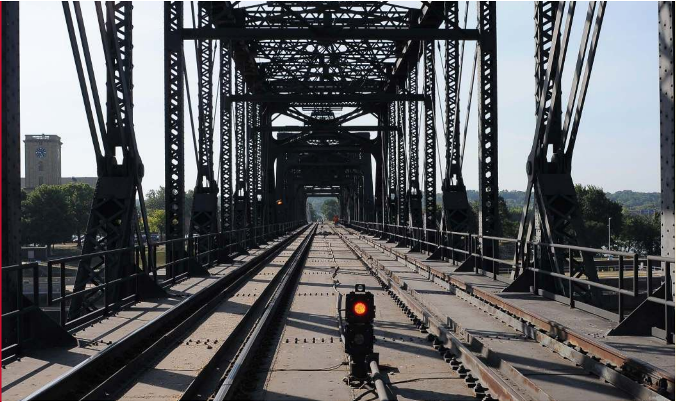
Existing Government Bridge | Source: HDR
