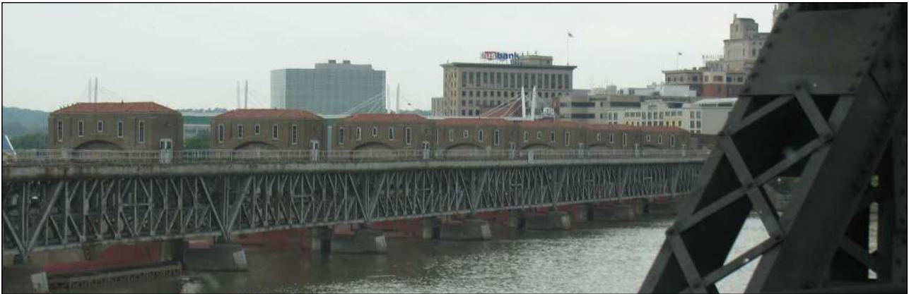
Existing Dam 15 from Government Bridge | Source: HDR
