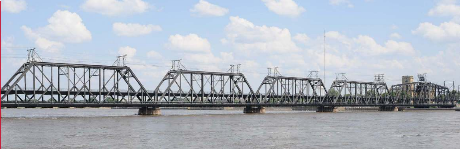
Existing Government Bridge | Source: HDR
