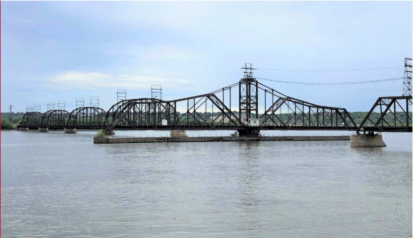
Existing Crescent Bridge | Source: HDR
