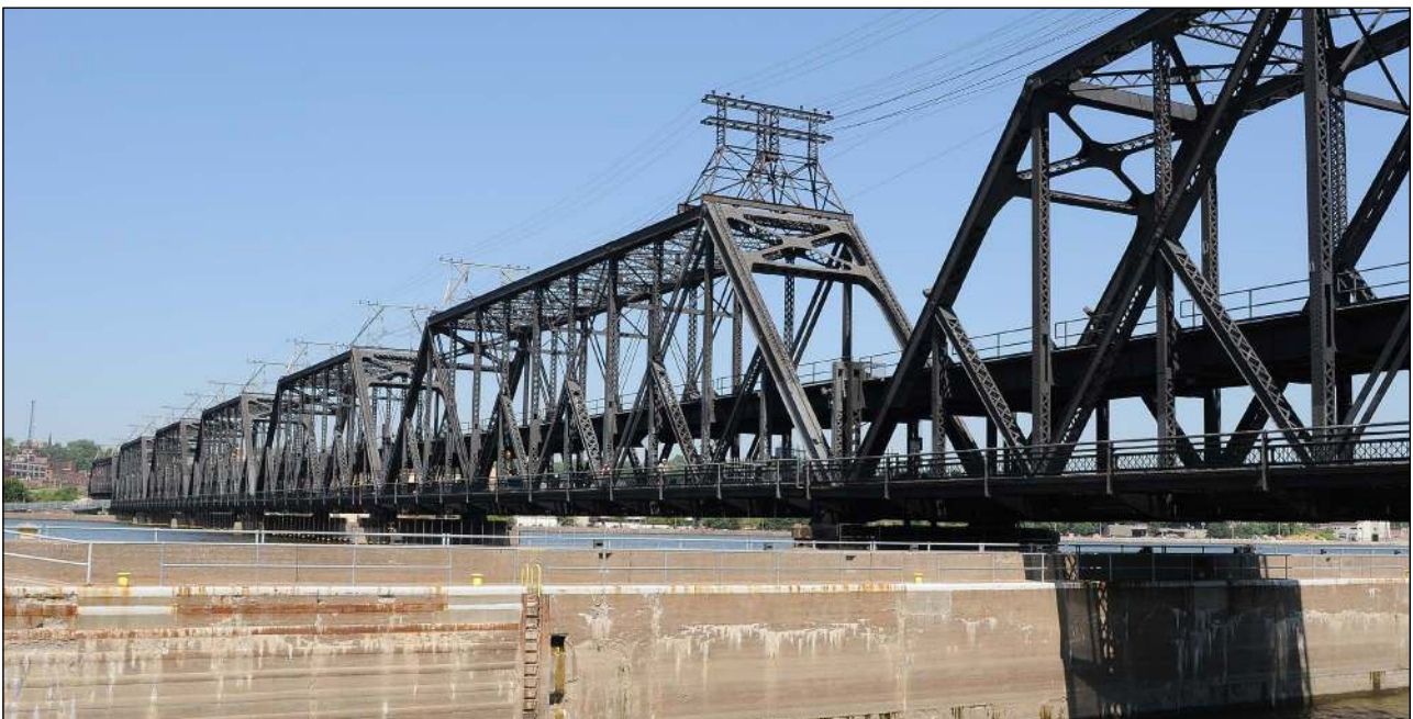
Existing Government Bridge at Lock 15 | Source: HDR
