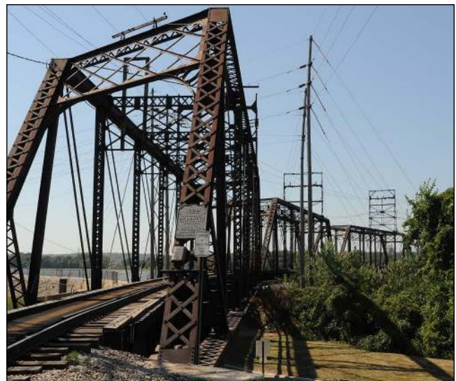
Existing Crescent Bridge | Source: HDR
