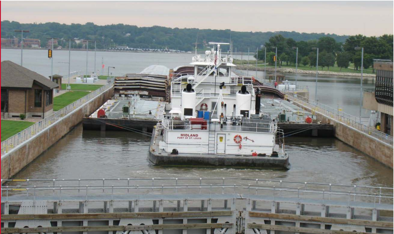
Barge Service at Lock 15 | Source: HDR
