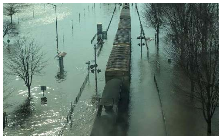
Figure 15: Flooded CP Track in Davenport, 2019
