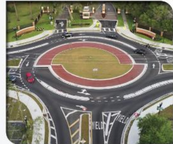
Source: Turbo Roundabout (Jacksonville, Florida), FHWA
