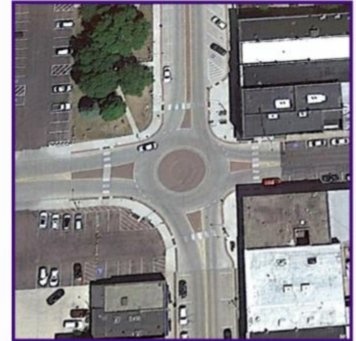
Highway 24 in St. James after construction, showing mini-roundabout, back-in angle parking, and improved crosswalks
