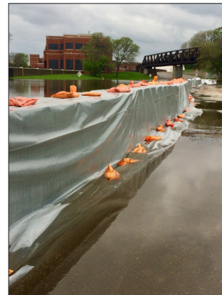
U.S. 67/River Drive, Davenport and Temporary Flood Barrier
