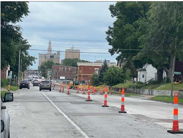
Figure 4.6 – Sample Road Construction, Davenport, Iowa
