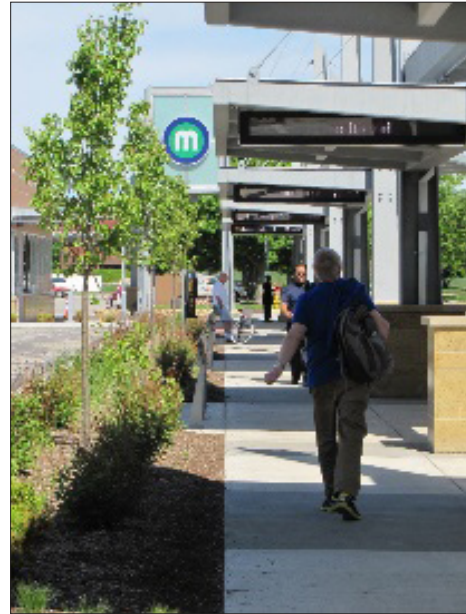
Figure 4.7 – MetroLINK District Station, Rock Island
